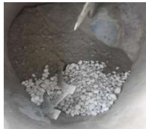
Fig.2: Mixing of concrete ingredients
