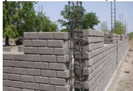
Figure 2): Confined DSM
