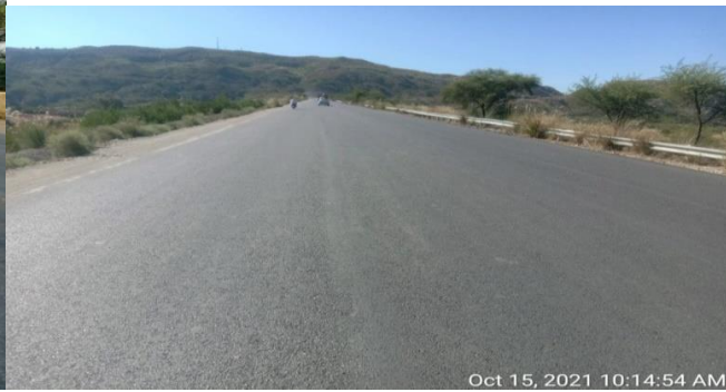
Fig: 5 Condition of road after 6 months (Revised JMF this Research) 1 layer of ABC (8cm) class A & 1 layer of AWC (5cm) class B
