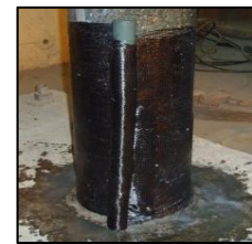
Fig.1 Loading Mechanism Fig.2 Damaged Pier Fig. 3 Prepared Surface Fig. 4 CFRP Application
