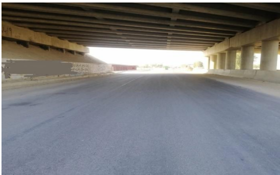
Fig: 2 No sign of Rutting underneath bridge (N-55)
