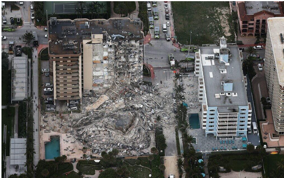
Figure 1: Aerial Photograph of Partially Collapsed South Champlain Tower [2]
